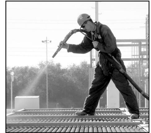
*Knight Industrial Services’ new bio-blast units are capable of up to 100 psi nozzle pressure, and are available as fully mobile units.*
